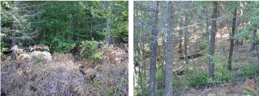
(Above Left, Katimiin Plantation Thinning Project before treatment.) Note the abundance of contiguous ground and ladder fuels. In this condition, plantations can experience excessive mortality during wildland fires and are not readily accessible to many wildlife species.
